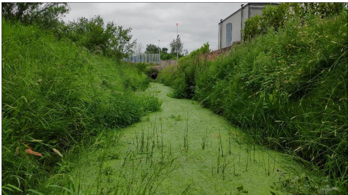
Plate 8.6: Representative image of site 1A (facing downstream towards road culvert).
