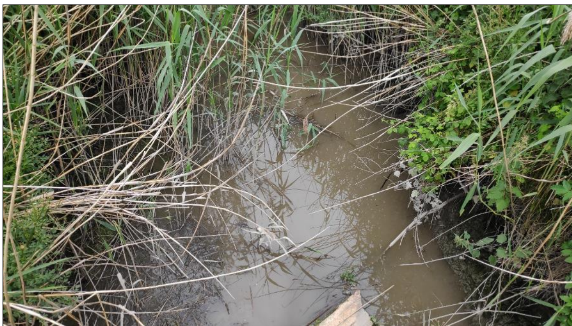
Plate 8.7: Representative image of site 1B located at the culvert leading to Ballynaclogh River.
