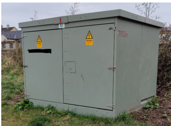
Figure 18.8: Sample ESB Kiosk Sub Station
